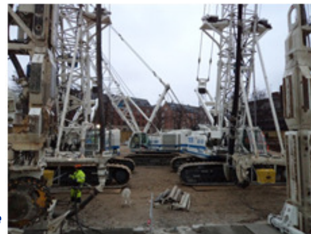
Copenhagen (DENMARK) CITYRINGEN work site
