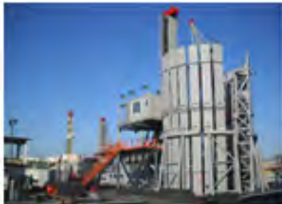
Hydraulic Drilling Rigs
