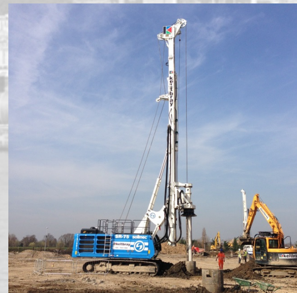
New state-of-the art Soilmec SR-75 in a UK work site
