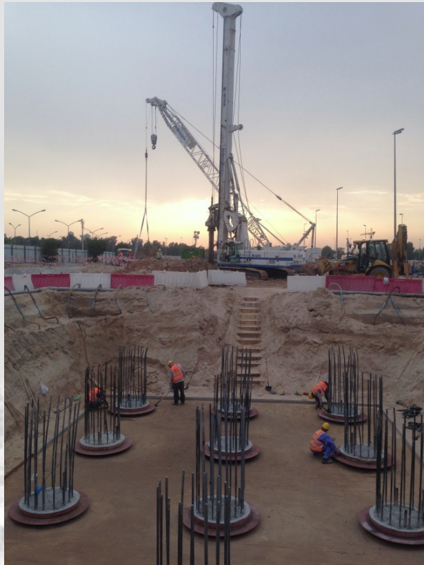
Soilmec foundation rigs
