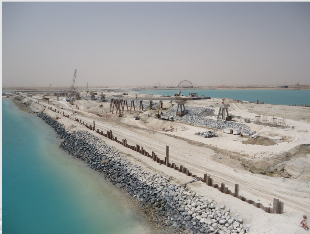
Soilmec SR-60 foundation rigs at work
