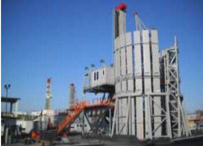
Hydraulic Drilling Rigs
