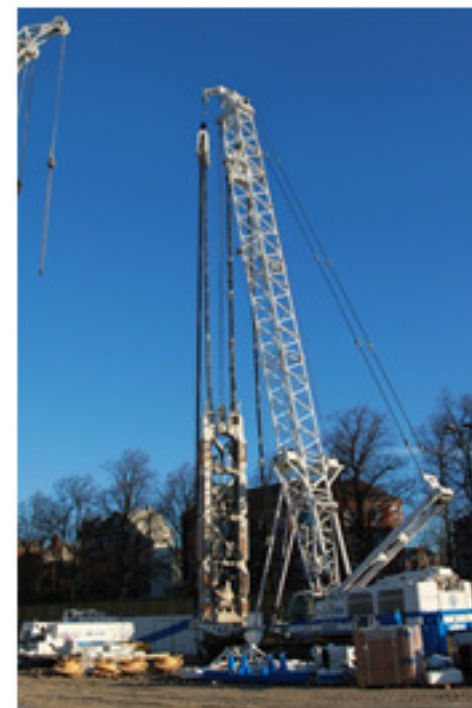
Copenhagen (DENMARK) CITYRINGEN work site
