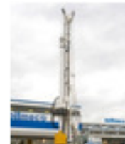
LARGE DIAMETER PILE
